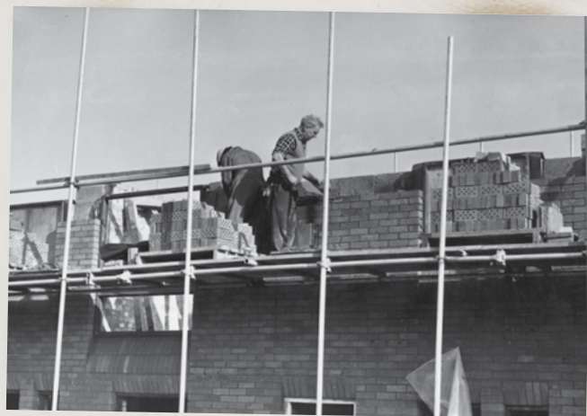
Bricklayers working on site in the 1960s
