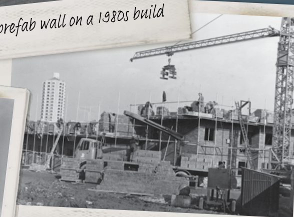
Building work in progress in 1971
