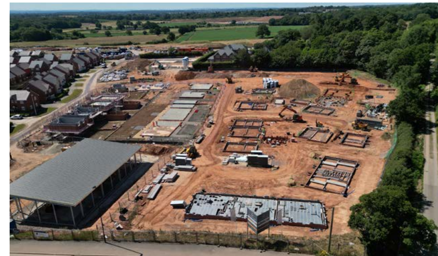
Work on site at Westwood Park, Burton Green - our first development to be run from the very start by the West Midlands office
